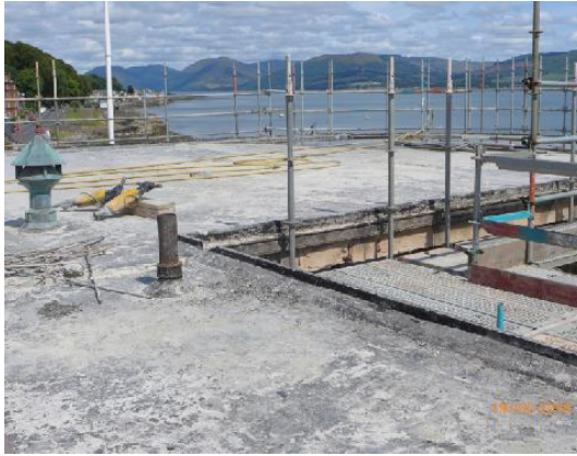
Existing roof finishes previously removed
