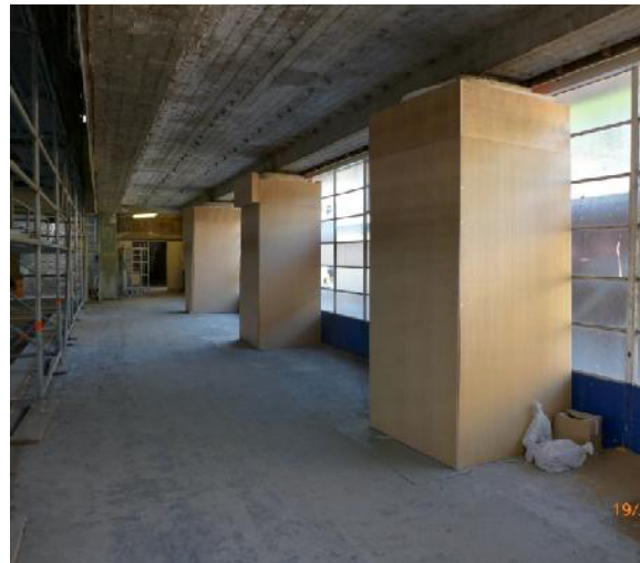
Upper Ground Floor – Protection maintained to the feature columns to the Main Hall.
