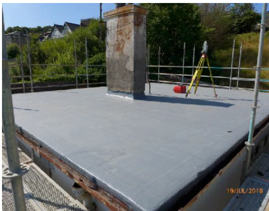
New roof covering installed.
