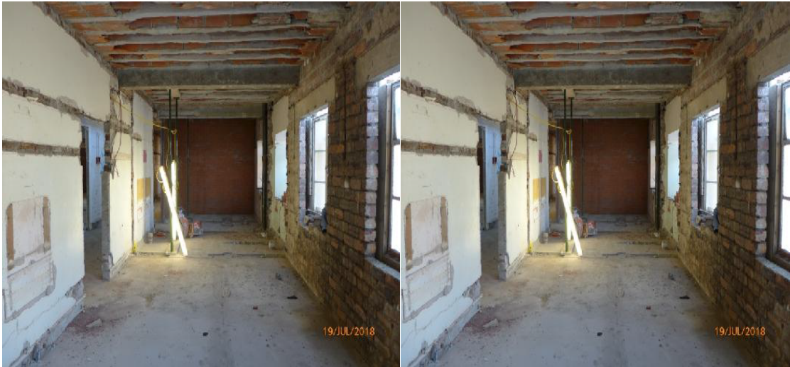
Upper Ground Floor – Back Stage Area.
