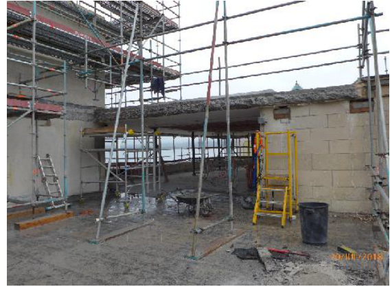
Removal of the overhang in progress.
