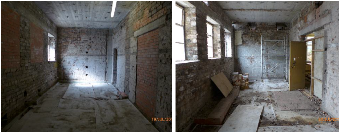
Upper Ground Floor - Existing ladies and Gents WCs next to main stair.
