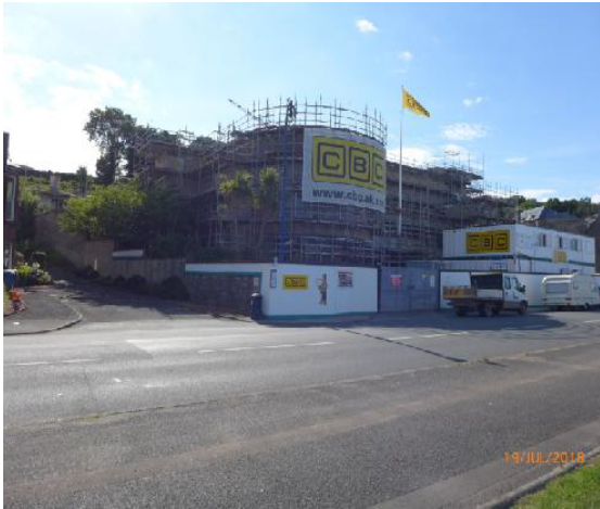
South and East Elevations
