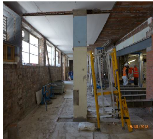
Lower GF – Looking South from existing Gents & Ladies WCs
