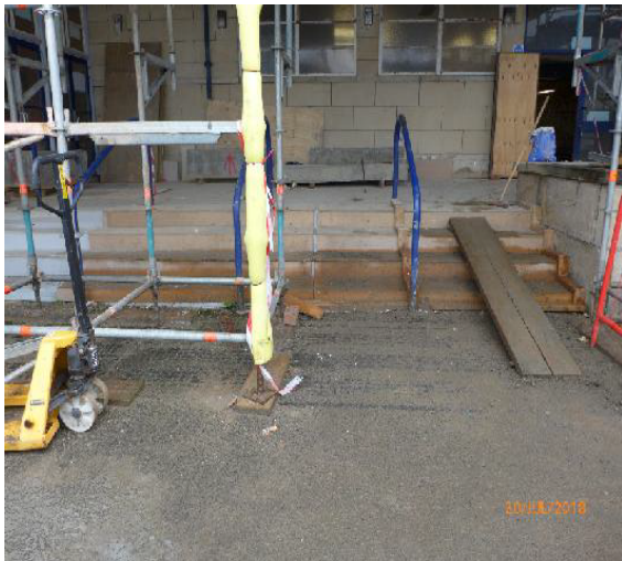
Front Entrance Steps – Protection Maintained.
