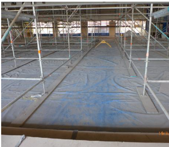
Upper GF – Protection maintained to the floor of the Main Hall
