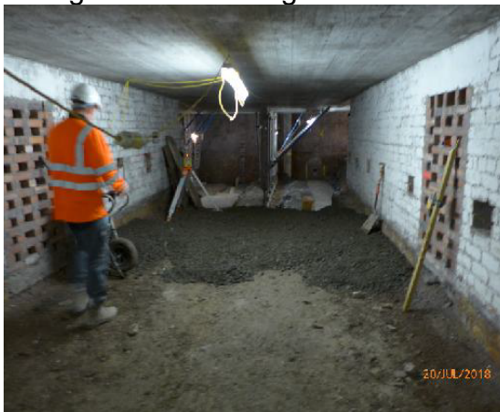
Auditorium Undercroft – Hard core subbase for new ground bearing slabs in progress.
